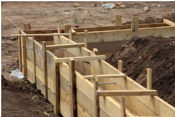
Figure 3: Wood formwork ( www.construire.it )
