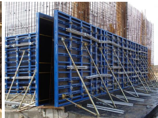
Figure 4: Metal-plywood formwork ( www.ceta.it )
